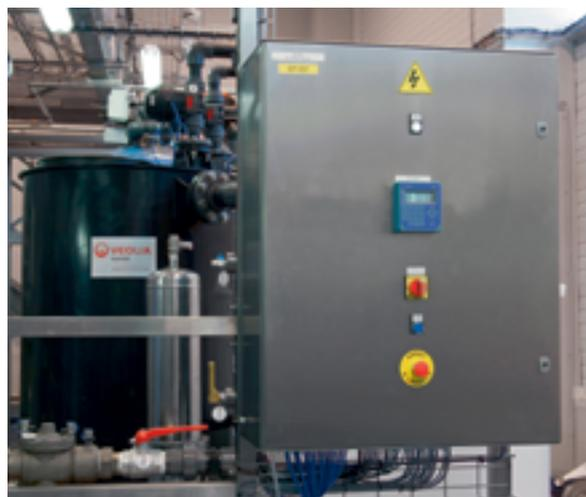
The conductivities are monitored on WFI loops by multiple METTLER TOLEDO Thornton transmitters including the 770MAX. The 770MAX is coupled with the 5000TOC analyzer which measures a USP critical parameter: total organic carbon. “METTLER TOLEDO Thornton’s ‘Smart’ sensors give us peace of mind for the commissioning phase; particularly the automatic ‘plug-and-play’ sensor setting recognition,” emphasizes Hervé Caron.
