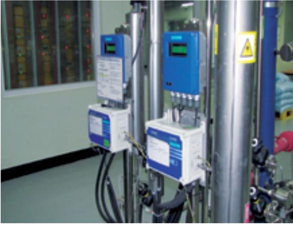
Control panel shown with Thornton 770MAX transmitter and 5000TOC sensors
